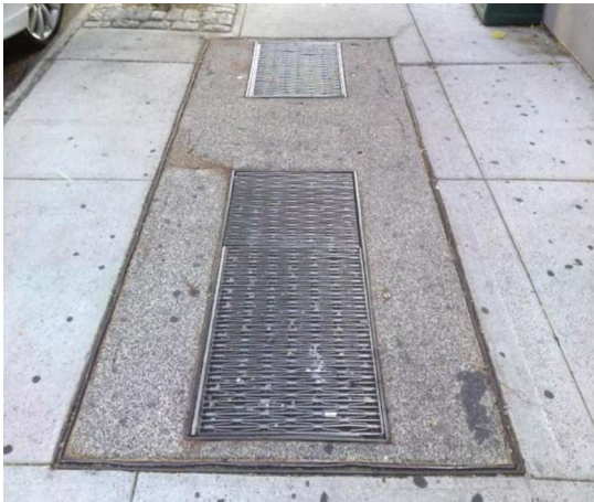
Fig. 4. Underground vault below sidewalk, containing Transformer 1.
